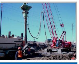
**Dry Bottom Feed Stone Columns** Increase cyclic shear resistance and bearing capacity of silty sands that will bear the MSE wall.
